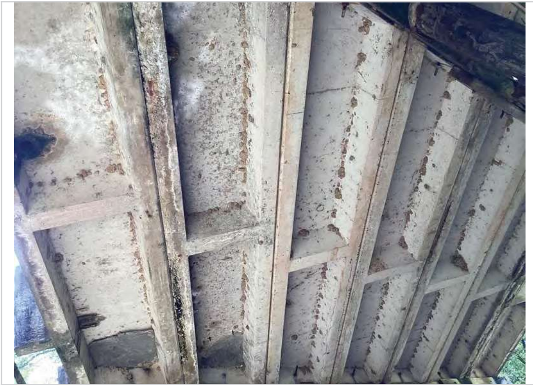
Bottom deck span #4
