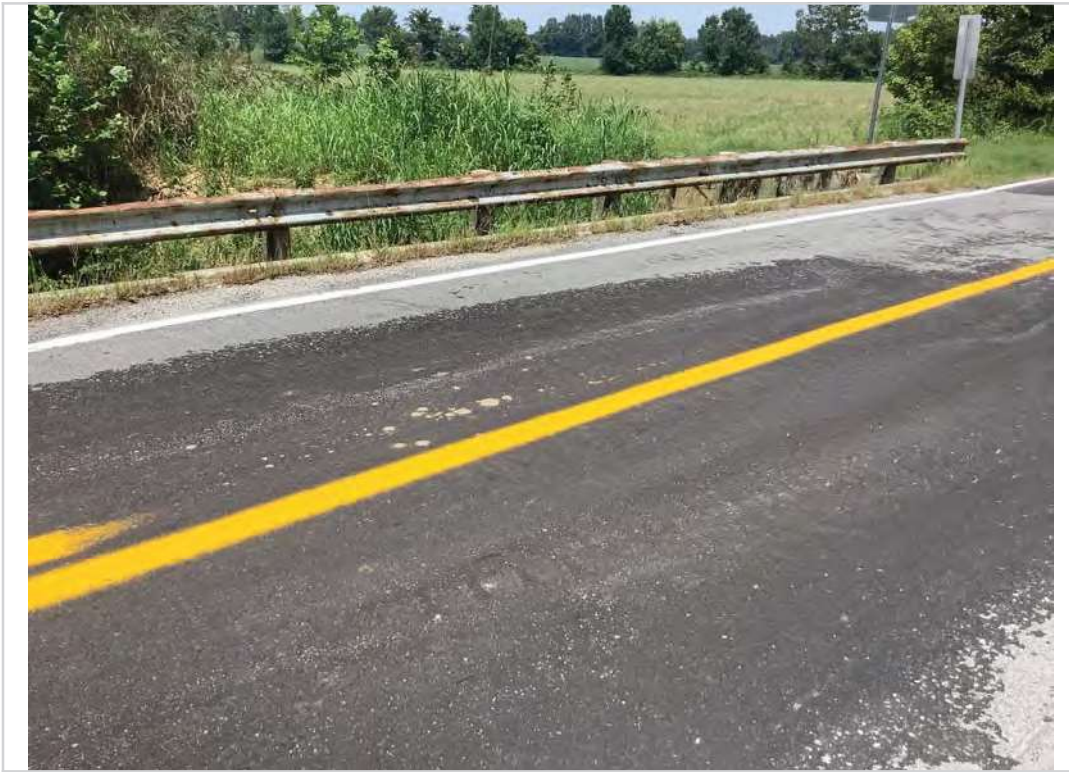
Span 3 view across top deck
